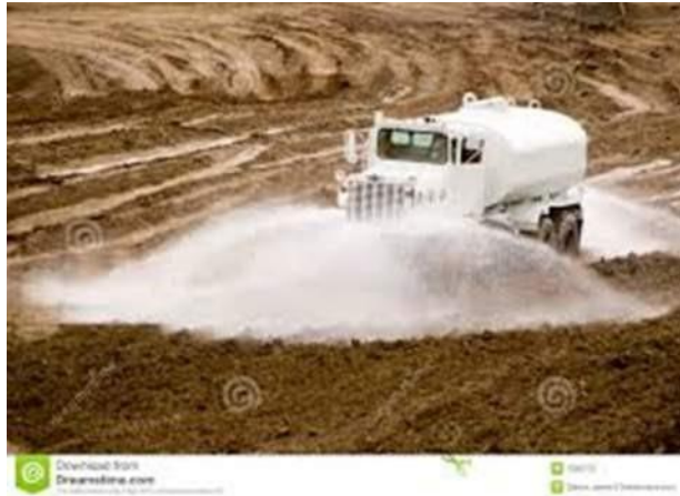
Figure 5.2: Dust Control Water Trucks (Illustrative Only)
