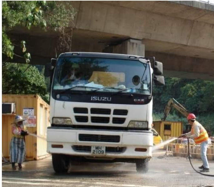
Figure 5.4: Trucks Being Washed Before Leaving Work Zone (Illustrative Only)
